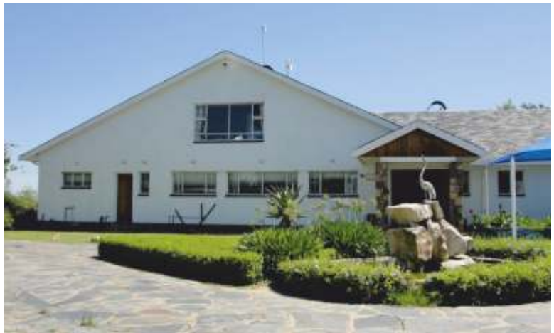
The Professional Aviation Services Office at Lanseria Airport
